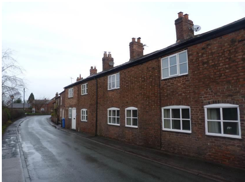
Terraced cottages on Woodhouse Lane
