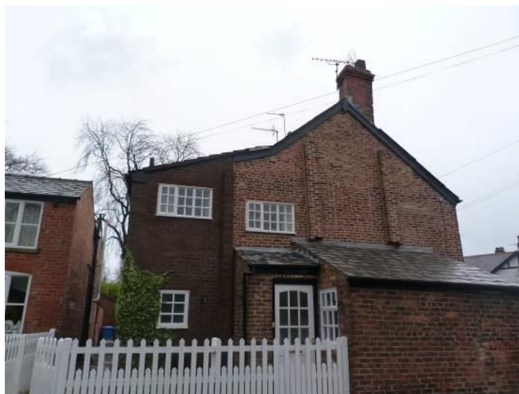
End elevation of Rose Cottage
