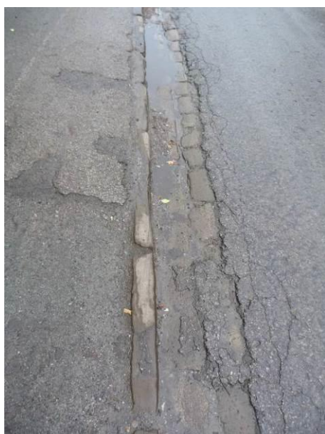
Historic curb stones and cobbled gutter
