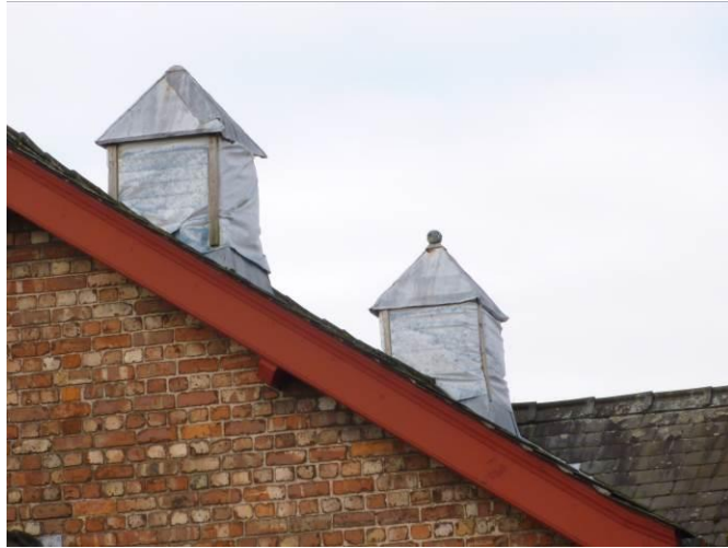
Sheeted ventilators to Village Farm out-buildings
