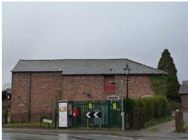
Substation in the centre of the village
