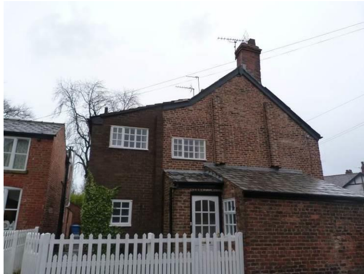
End elevation of Rose Cottage
